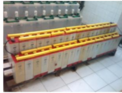
Gambar 3.2 Baterai Back Up Daya
