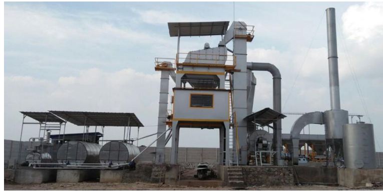
Gambar 1. Asphalt mixing plant
