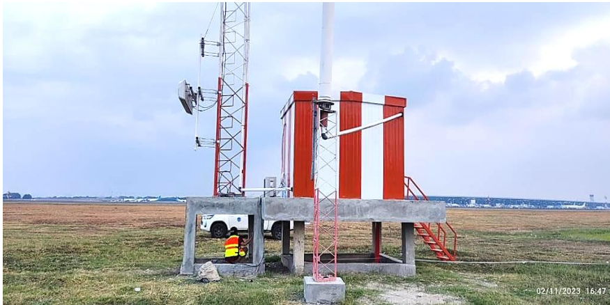
Figure 2. ILS GP Equipment Installation on Runway 24
